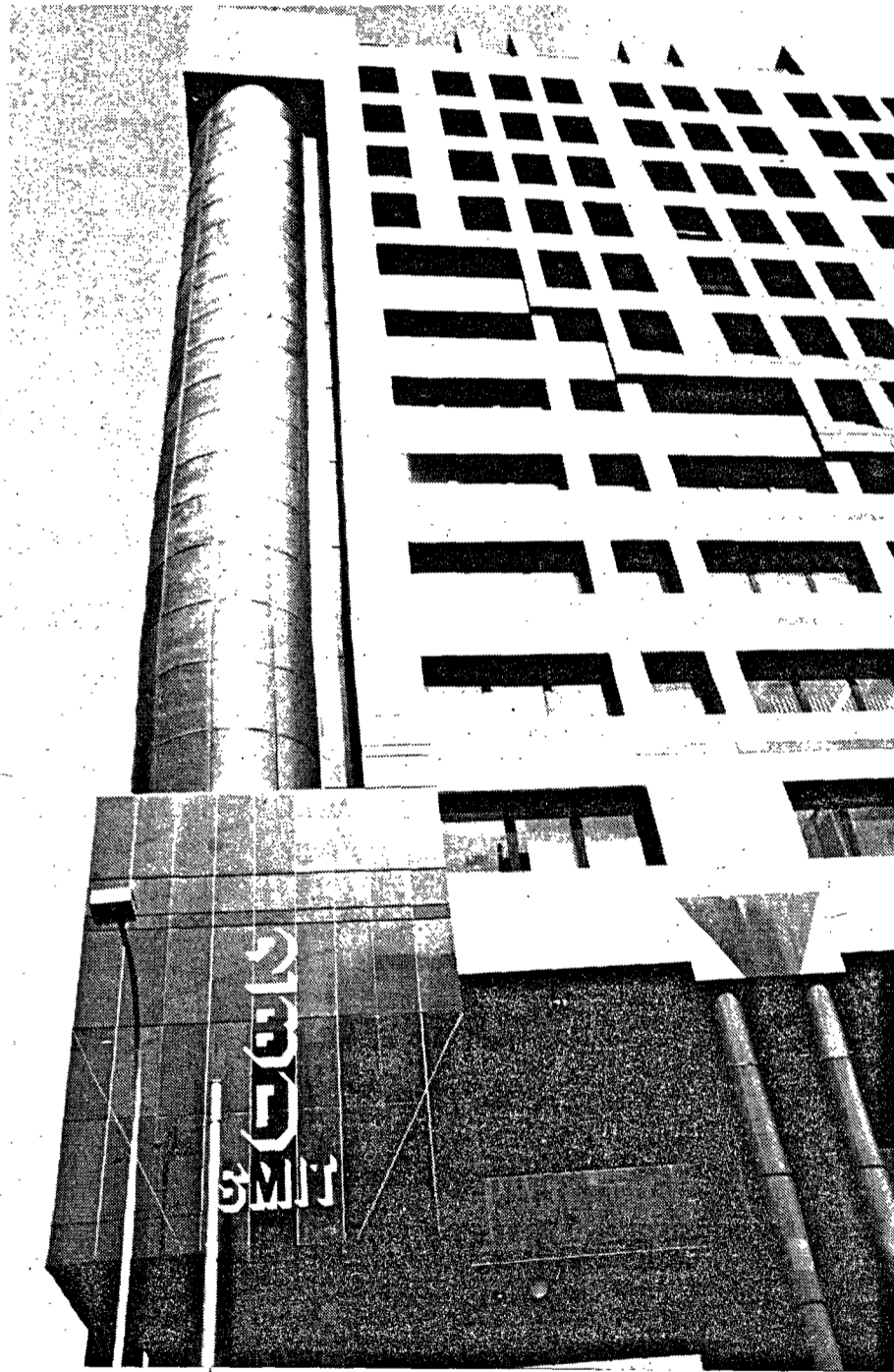
The recently completed Johannesburg headquarters for the Department of Posts and Telecommunications. (Photo's: Rodger Bosch.)
