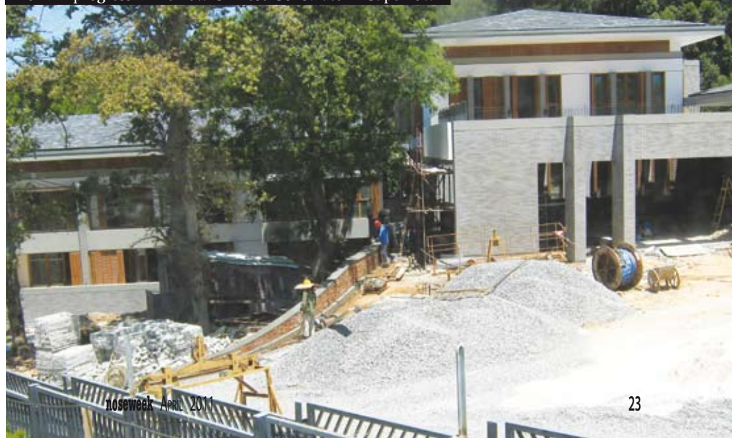
Work in progress... The new Chinese Consulate in Cape Town
