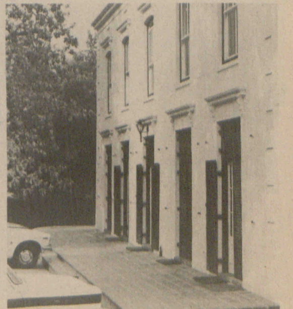
... are replacing the old.
