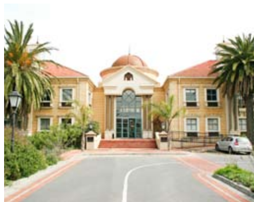
The Fidentia building in Century City, Cape Town.
