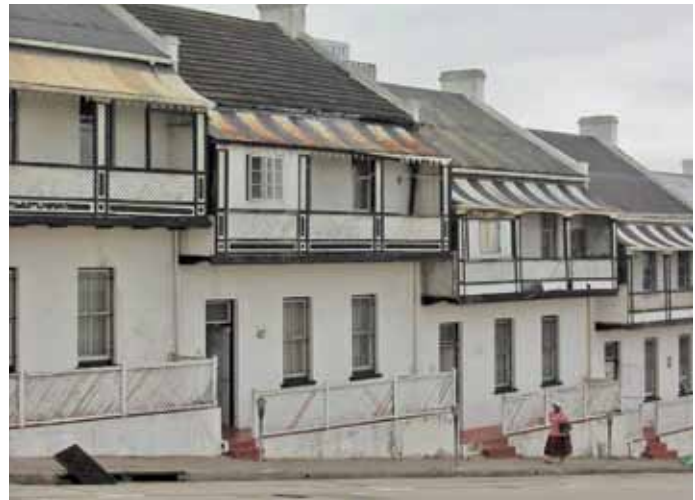
Donkin Street terrace before renovation
