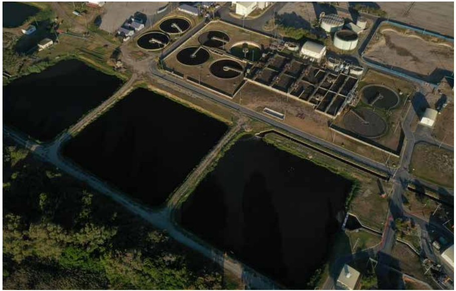
Potsdam water treatment plant
