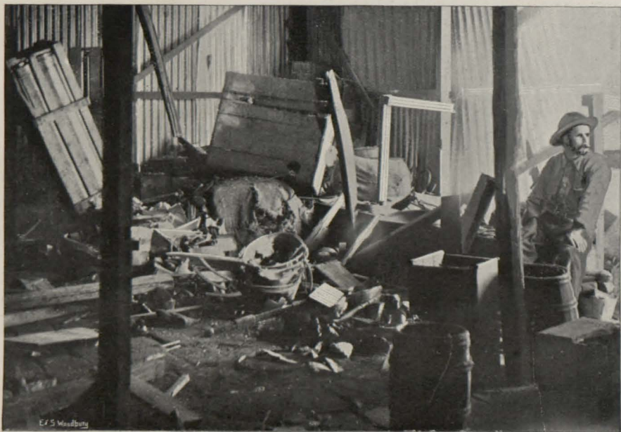
SHELL DAMAGE, WHITELEY WALKER'S STORE.
