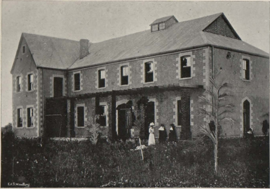
THE CONVENT, SHOWING SHELL DAMAGE.
