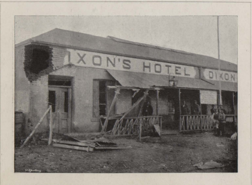
DIXON'S HOTEL, SHOWING SHELL DAMAGE.
