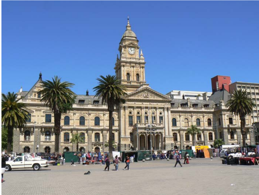
Figure 8: Picture of the City Hall of Cape Town. The carillon is installed in the area below the clock.
