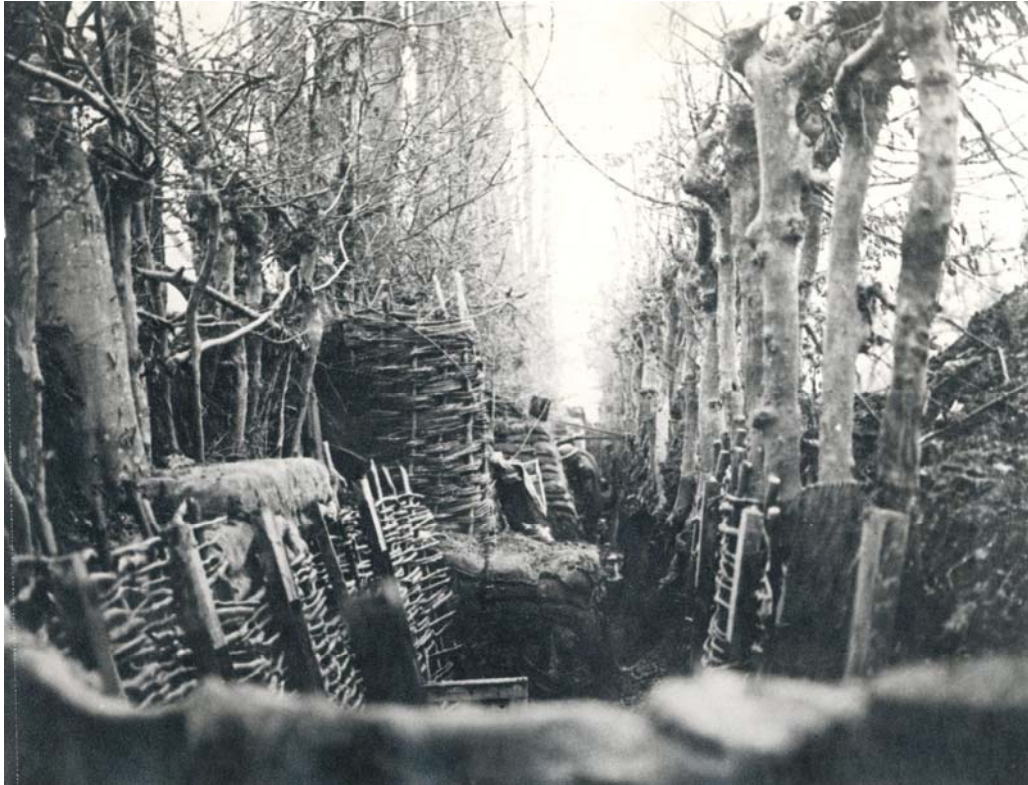
Figure 3: Picture of a concealed trench in the Great War.
